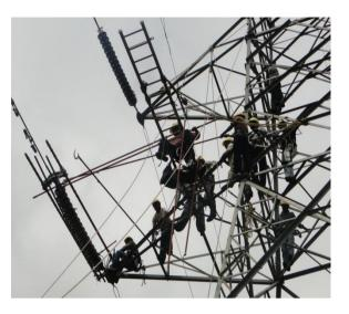
Fig.12: Changing of insulators on 220 KV Dead End [10].
